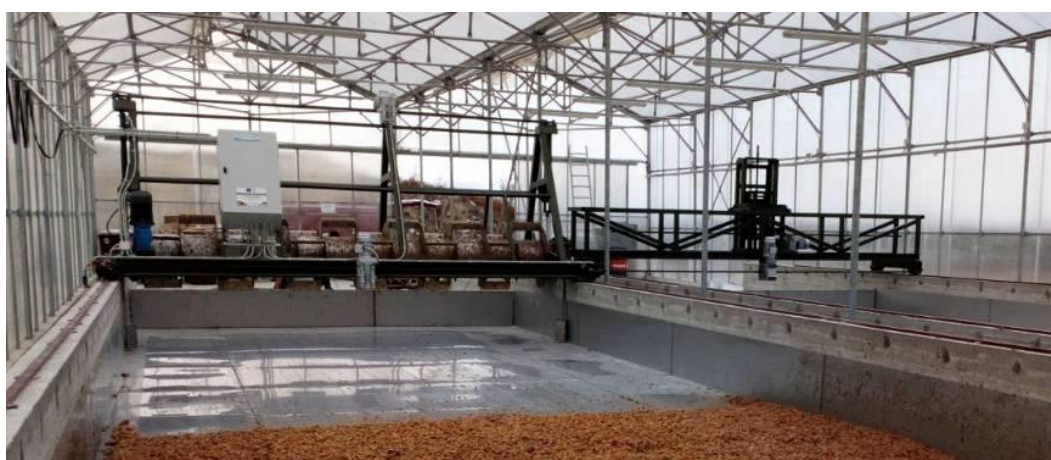
Picture 4. The turners into the drying unit of the F4F pilot unit. Under the inox drying halls there is the thermal drying system
