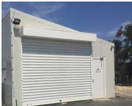
Picture 5. Automatic mechanisms in the doors
