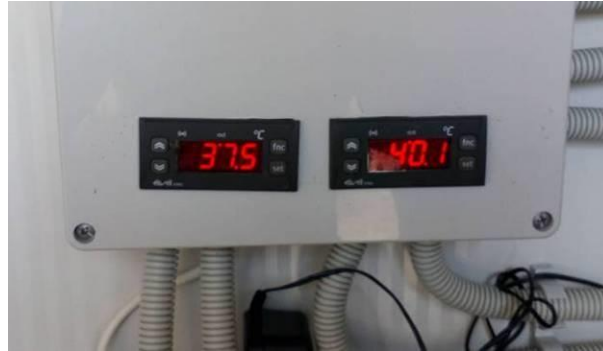
Picture 19. Temperature indication for both solar drying halls
