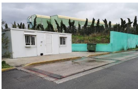
Picture 4. Weighbridge in the bio-drying MSW unit and weight recording unit
