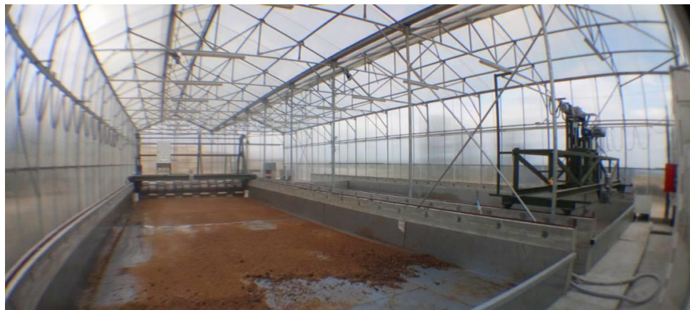
Picture 10. Panoramic view from the inside of the solar drying unit with the drying systems
