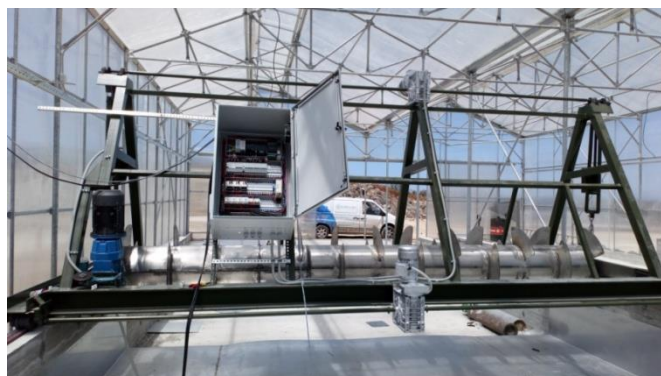
Picture 5. Placement of the electrical panel on the horizontal turner
