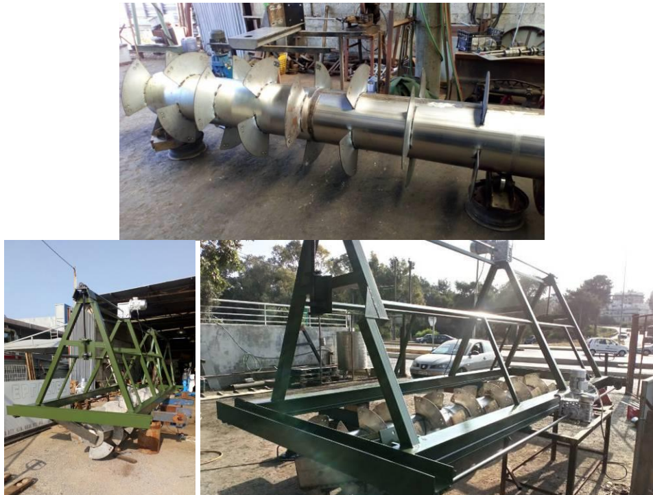
Picture 1. During the construction of the inox horizontal turner
