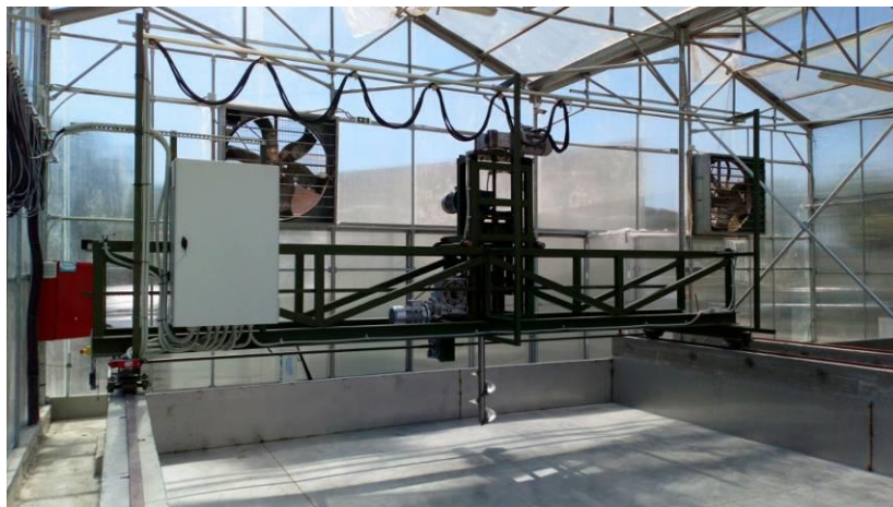
Picture 9. The installed vertical drying turning system on the drying hall
