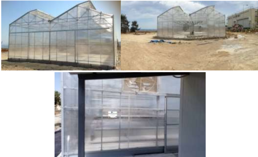
Picture 9. After covering the greenhouse with polycarbonate sheets
