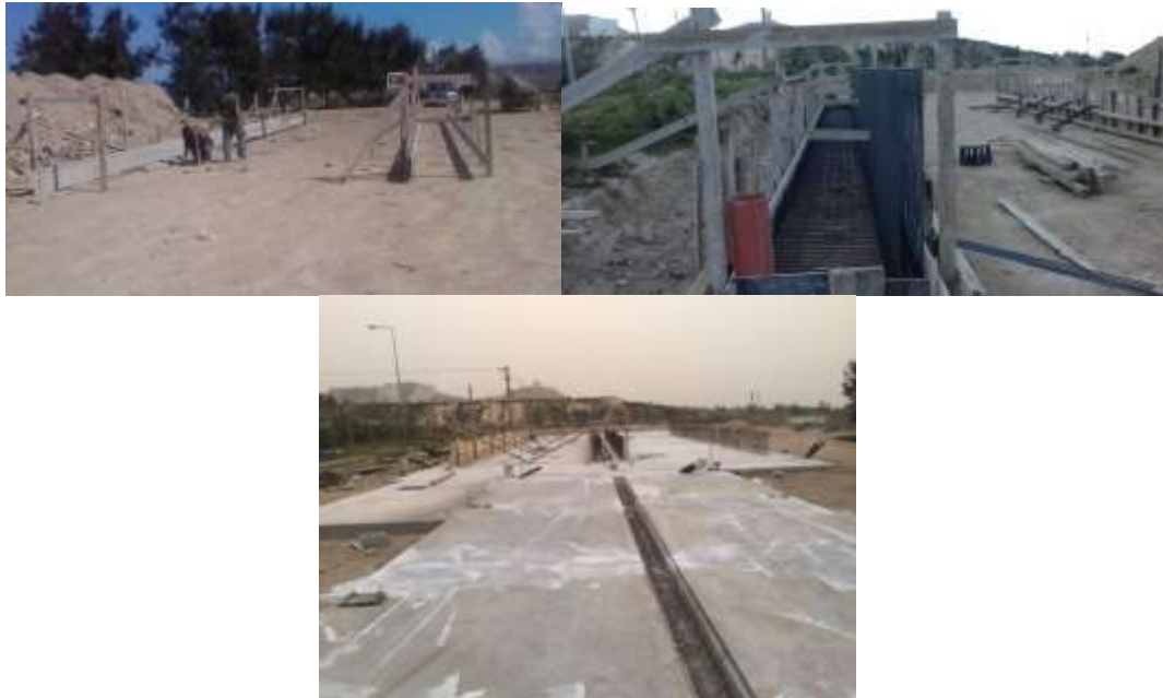
Picture 7. During concrete formwork
