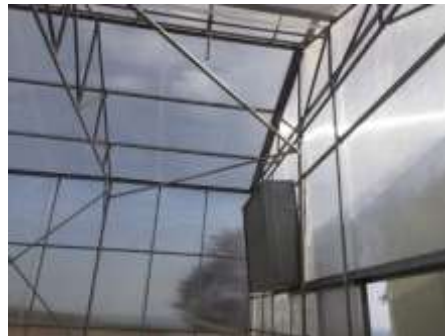
Picture 15. Fans into the solar drying greenhouse for air circulation
