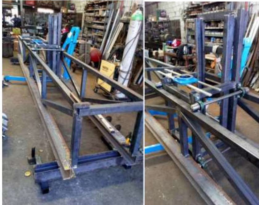
Picture 22. During the construction of the vertical drying system
