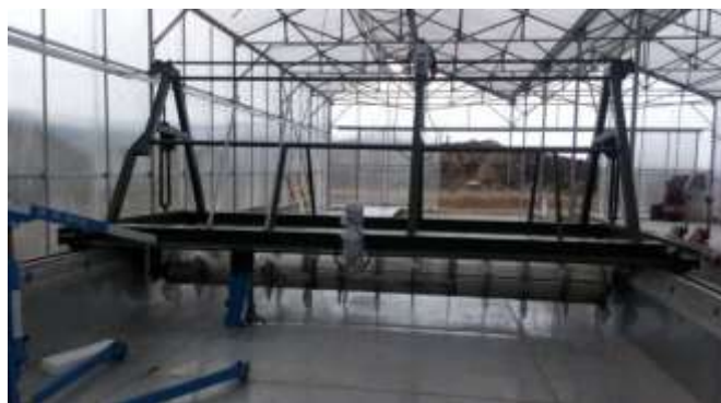
Picture 19. Placement on to the drying hall
