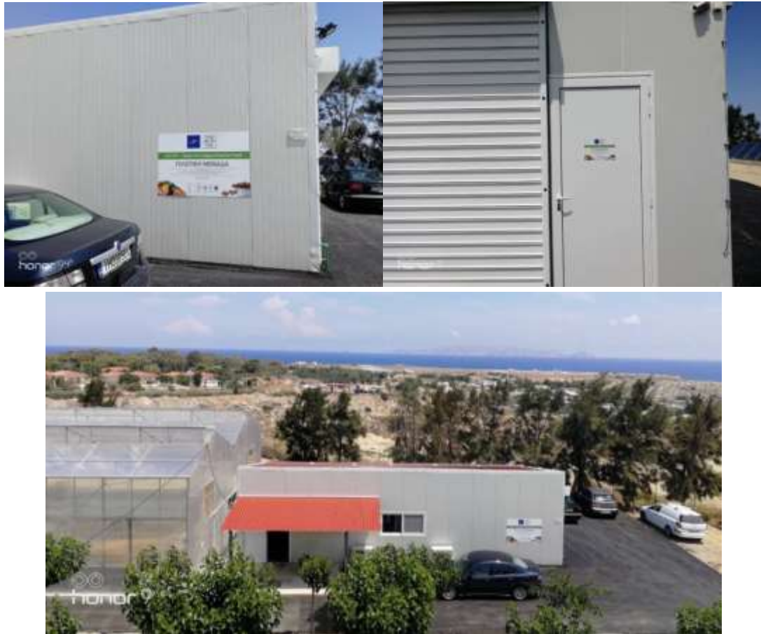
Picture 10. During the prefabricated unit construction with the relevant equipment
