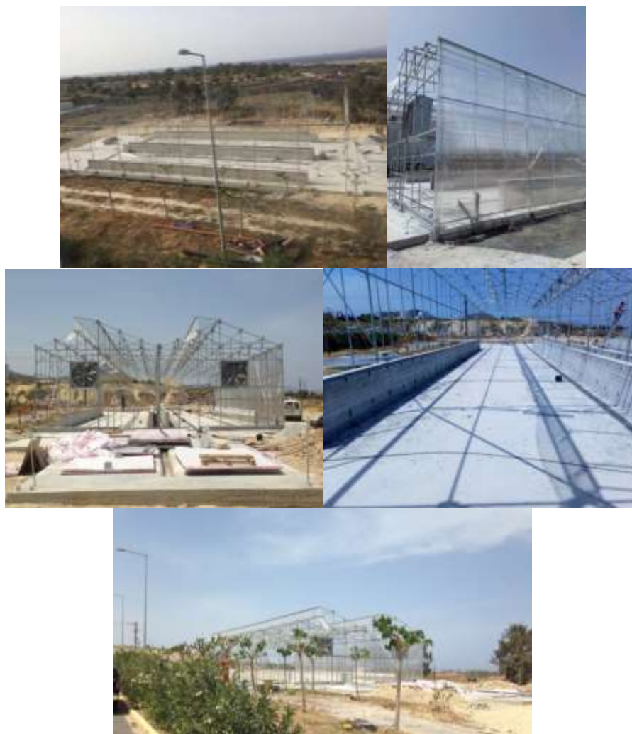
Picture 8. Construction of the greenhouse framework
