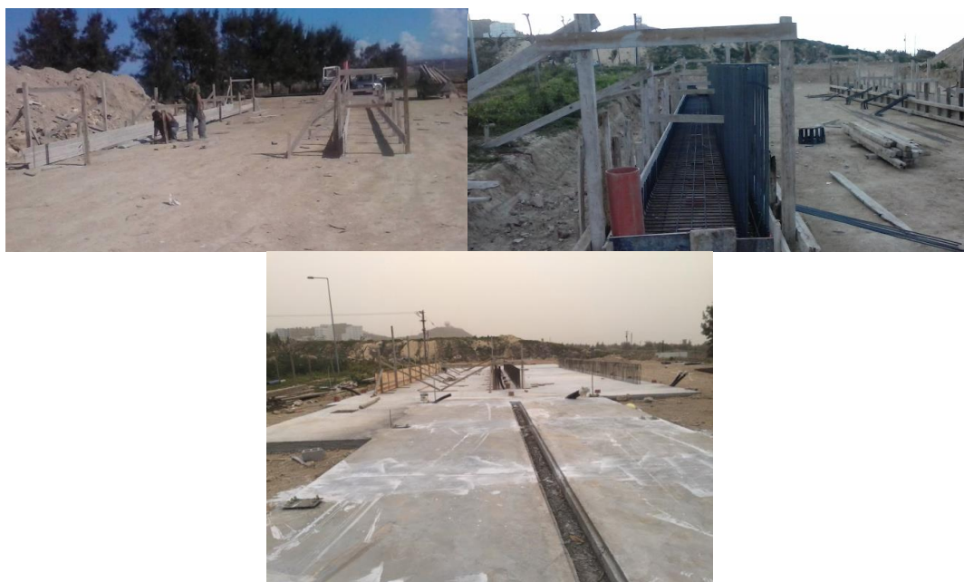
Picture 7. During concrete formwork
