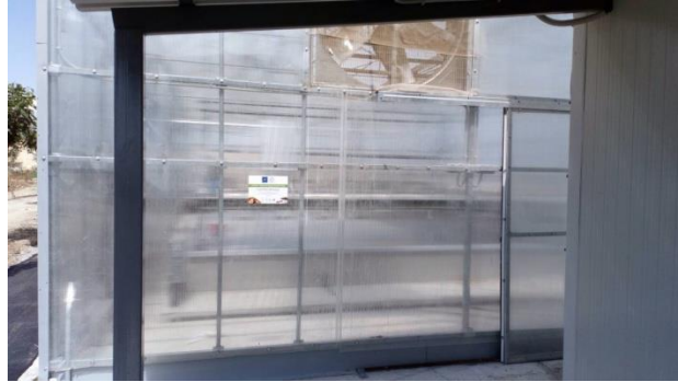
Picture 9. After covering the greenhouse with polycarbonate sheets
