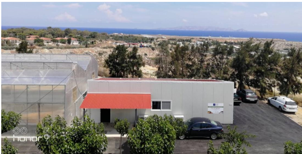
Picture 10. During the prefabricated unit construction with the relevant equipment
