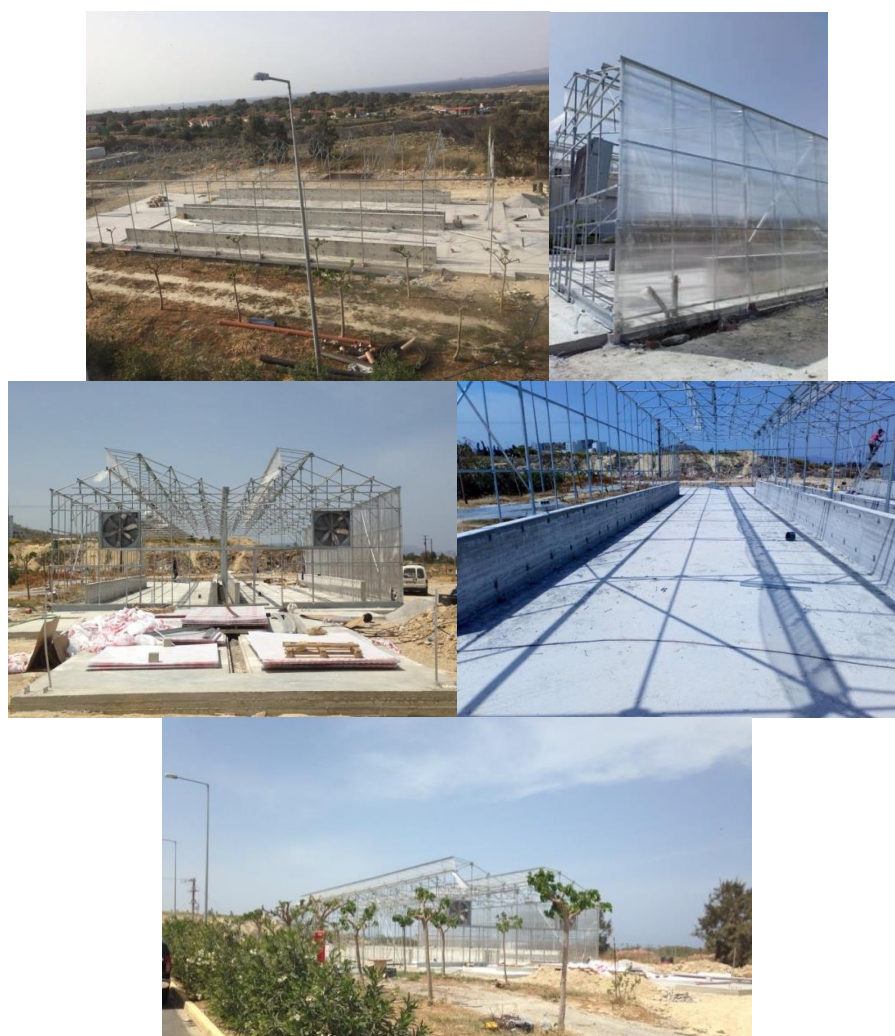
Picture 8. Construction of the greenhouse framework
