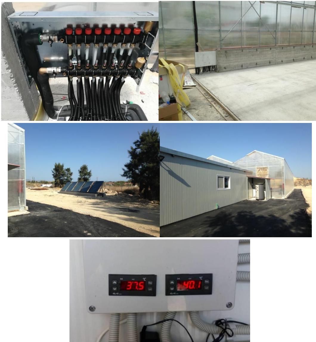
Picture 13. The heating system with the supply and return collectors, the boiler, the solar panels and the temperature display panel of the network of pipelines for the floor heating system
