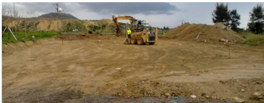
Picture 3. Works for grading the ground
